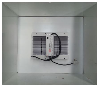
Step 4. Insert LED light engine into base plate and terminate to mains voltage.
