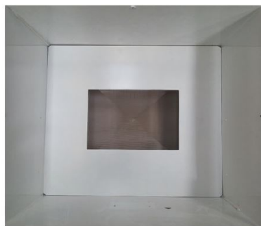
Step 3. Insert retrofit base plate.
